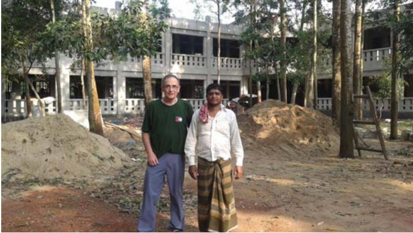
Moulvibazar, Bangladesh. Br. Eugenio Sanz (on the left) in front of the school which is under construction.
